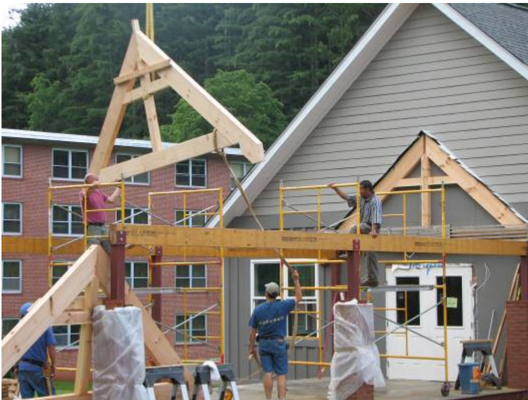
The crane helps out.
