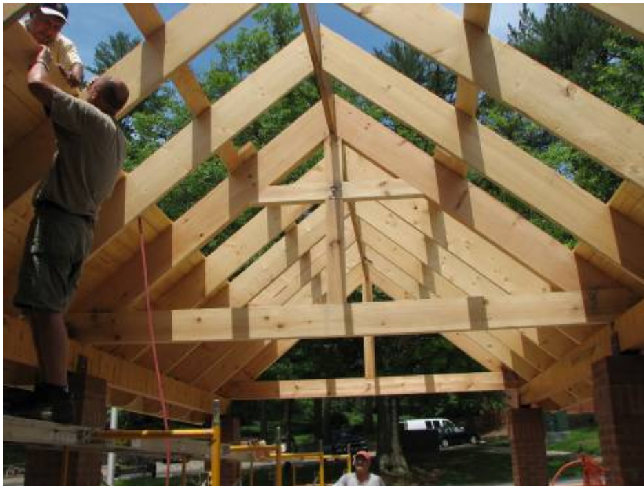
Joists are up and now the roof goes on.
