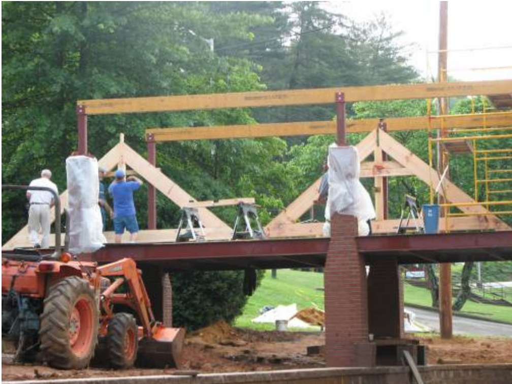
Notice the metal pillars wrapped in bricks.
