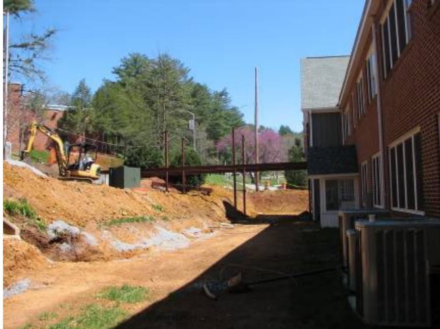
The steel for the Wesley Walkway is installed.
