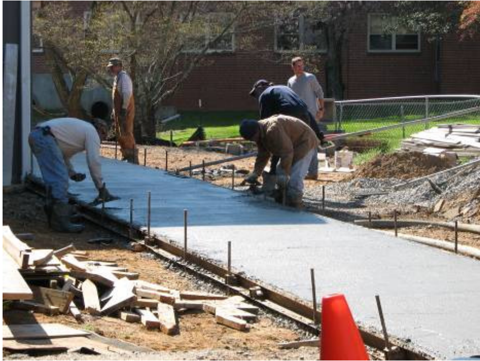
Sidewalks in the back of the church are poured.
