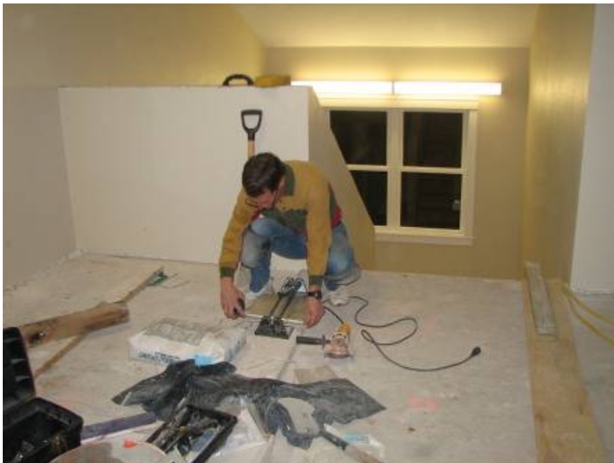
David C. cuts tile for the bathrooms.
