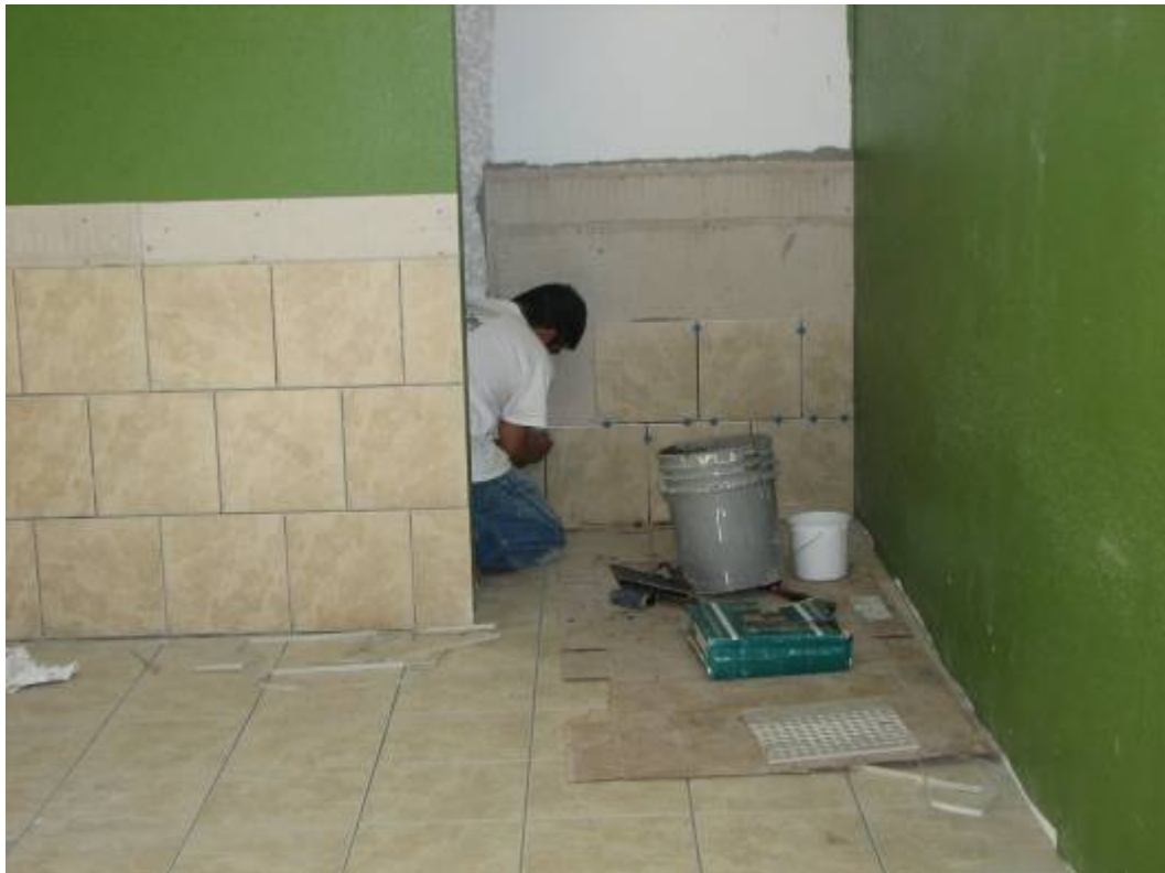
Grouting is next.
