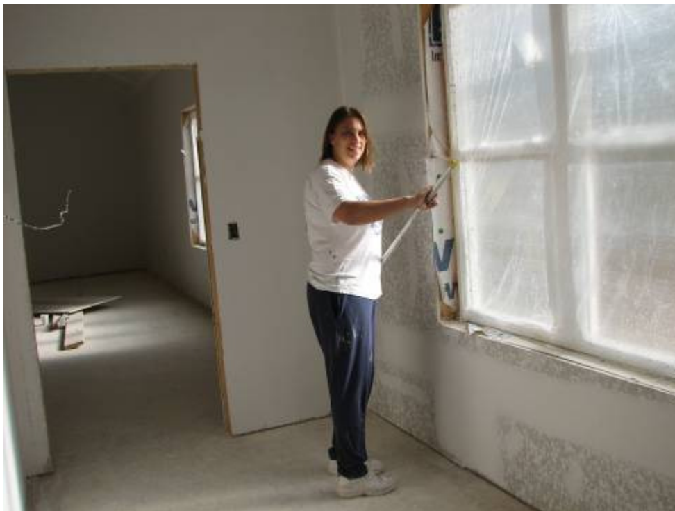
Julie painting in the kitchen of the new Wesley Center.
