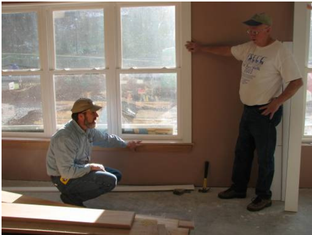
Tony and Earl check out the trim work installation.
