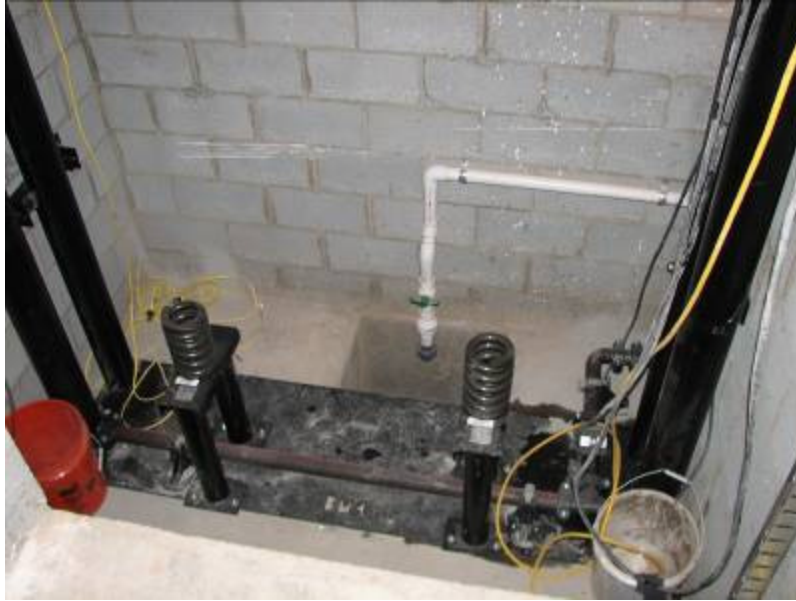
Looking at the guts of the new elevator shaft.
