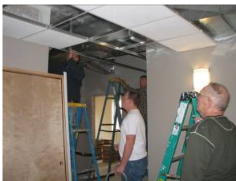
Installing the Drop Ceiling (Left) and Tiling the Bathrooms (Right)
