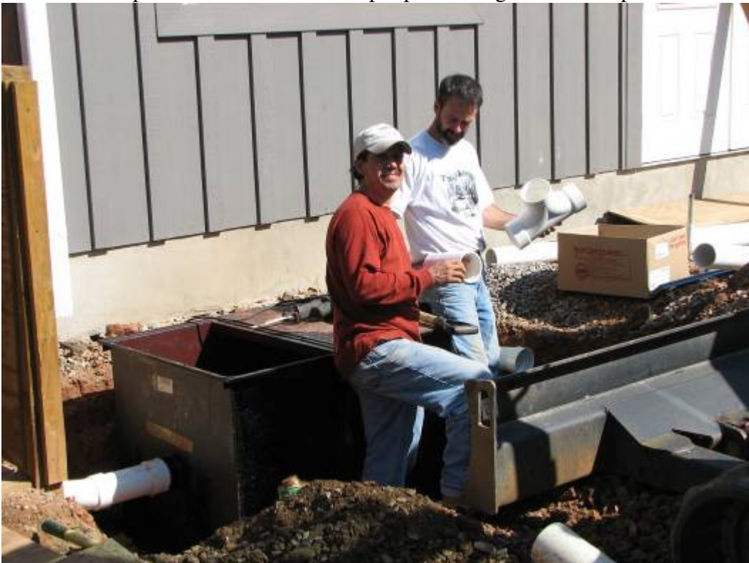
Our plumber Jason and his helper put in the grease interceptor.
