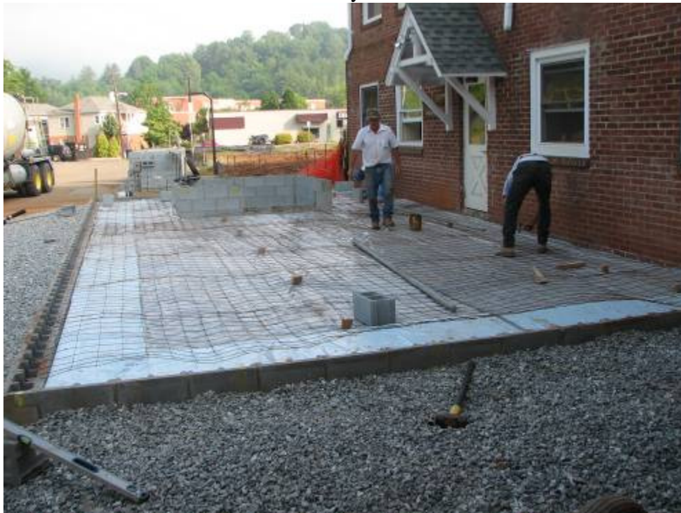
The slab for the new entry is readied for cement.
