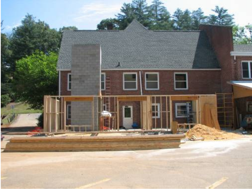
Walls for the new entry way start to go up.
