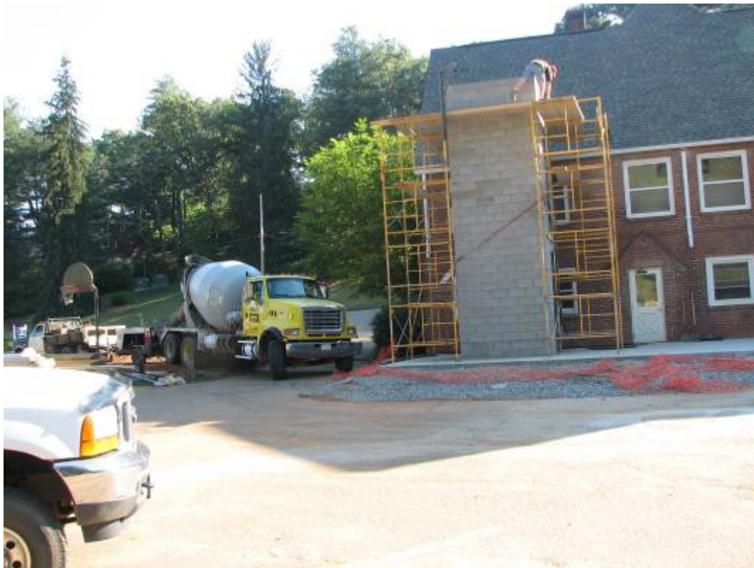
The elevator shaft is built.
