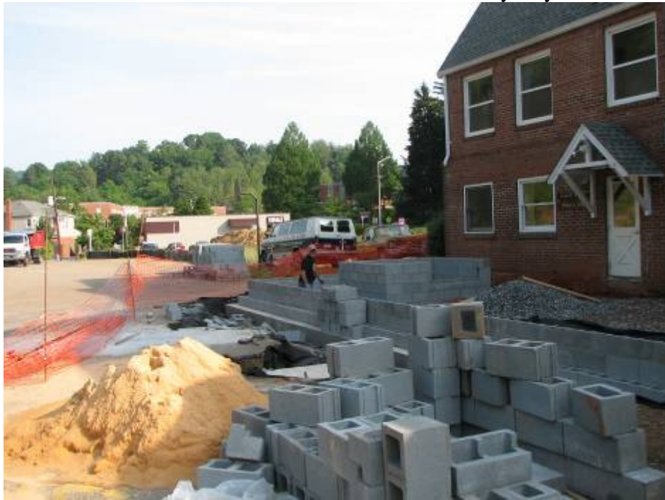
Block is laid for the foundation for the entry way.
