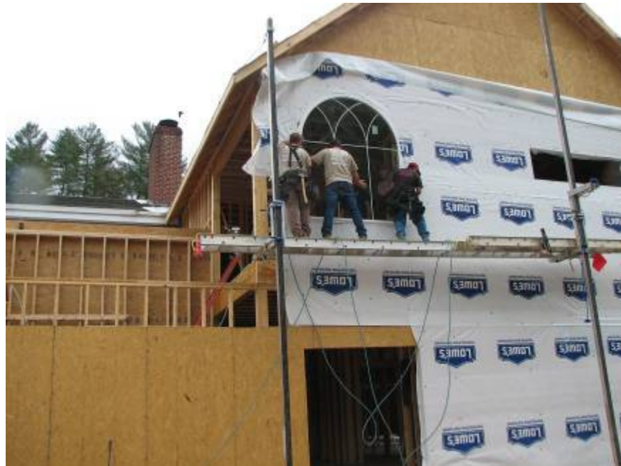
The high windows are installed by the framers.
