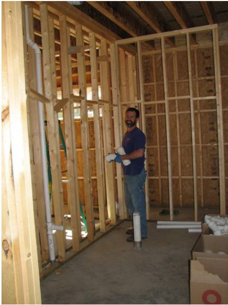
Rough plumbing is underway.
