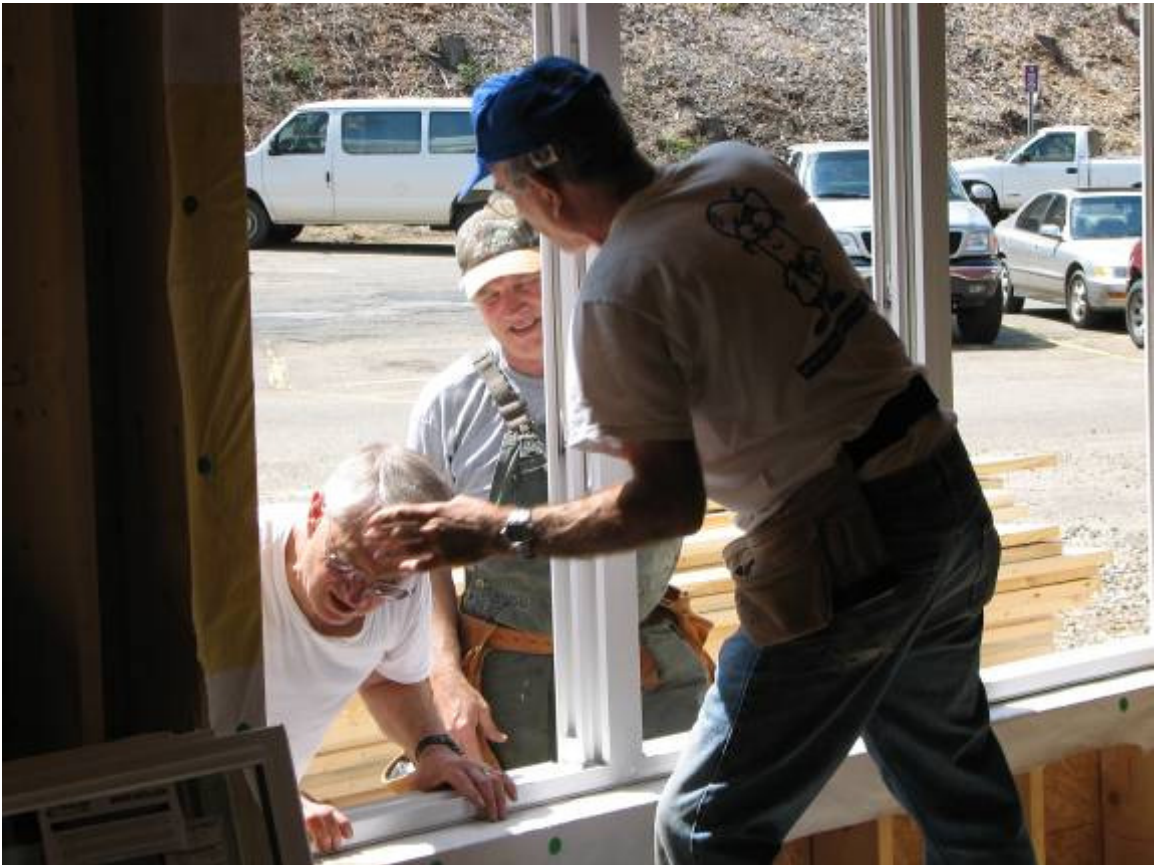
The low windows are installed by our volunteers.
