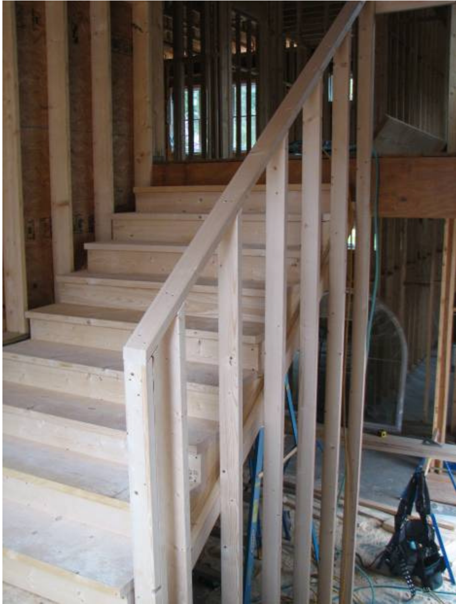
Stairs are built.
