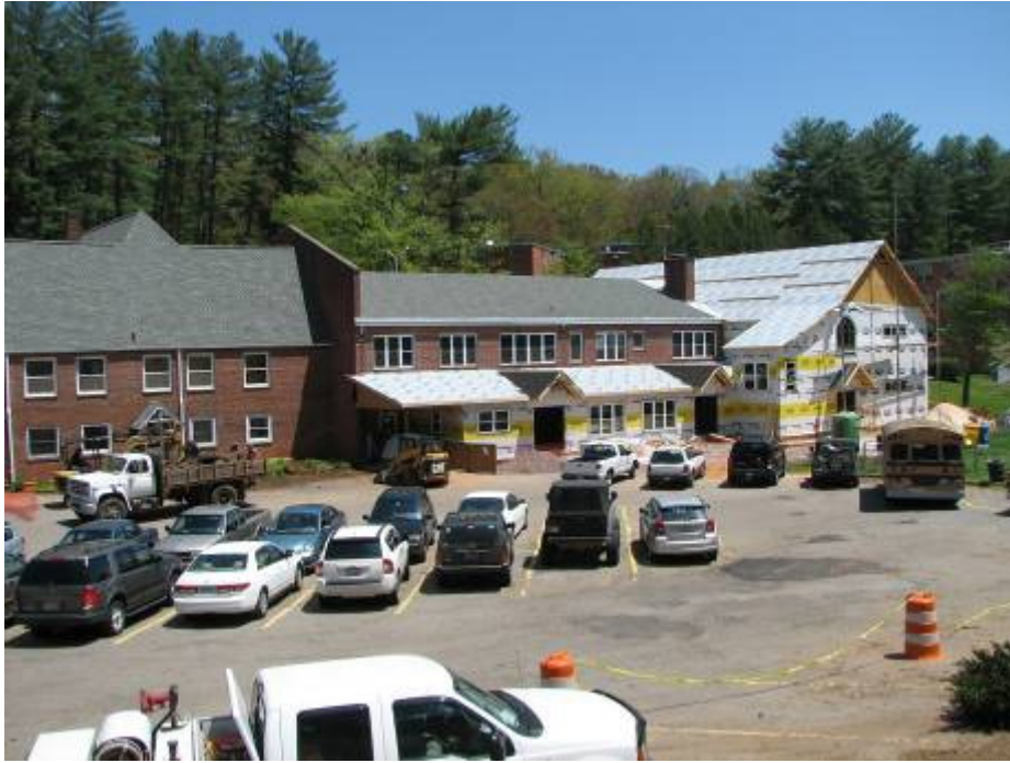
Framing for the main addition is done.
