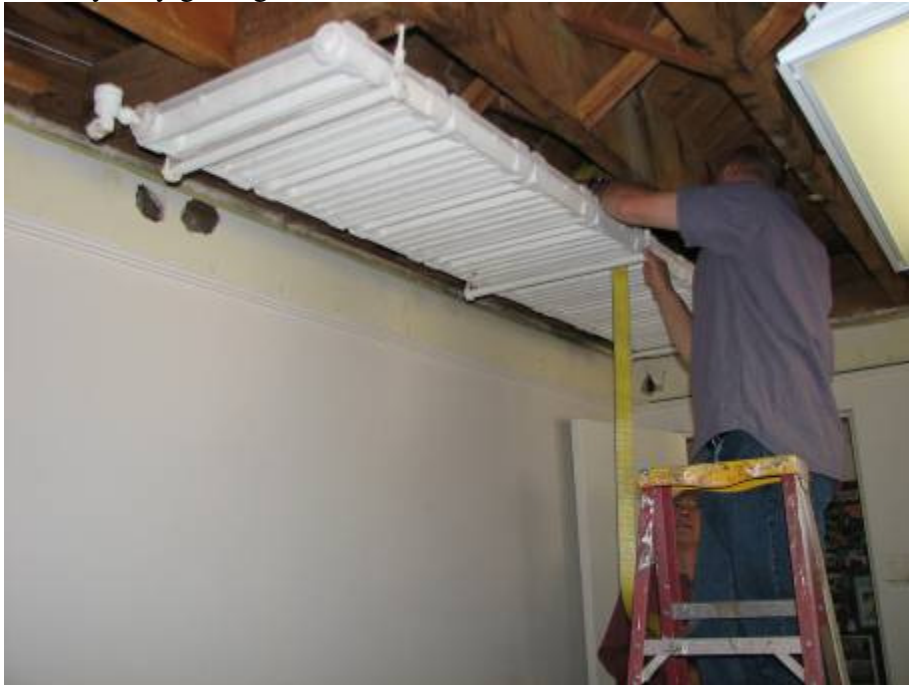
David uses a strap to secure the radiator before he cuts a section of it.
