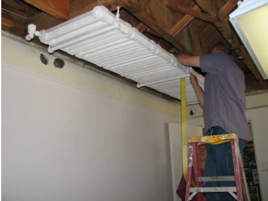
David uses a strap to secure the radiator before he cuts a section of it.
