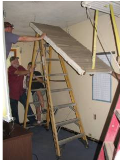
The radiators are lowered using a system of ropes. The radiator in the secretary's office (on the right) requires a little more ingenuity to get it down.
