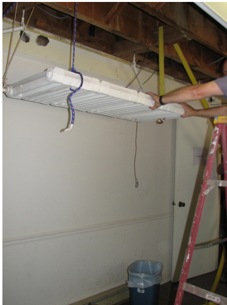
The radiators are lowered using a system of ropes. The radiator in the secretary's office (on the right) requires a little more ingenuity to get it down.
