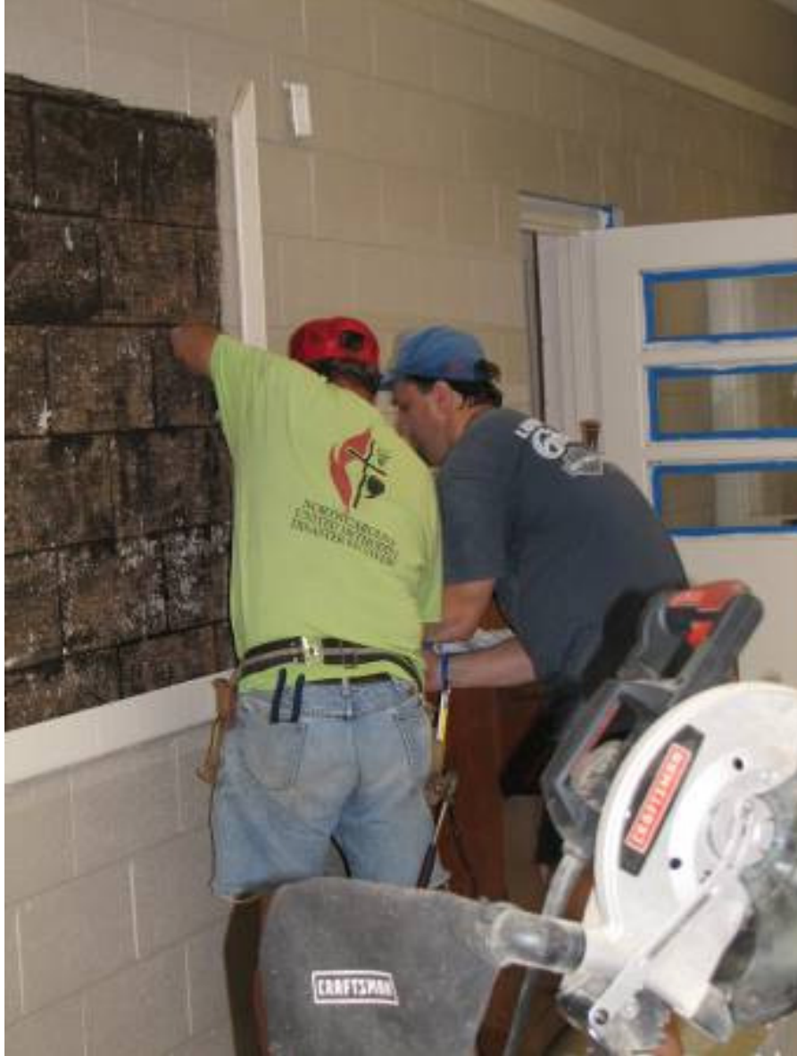
Lamar and Dean put up the trim for the new whiteboard and corkboards.
