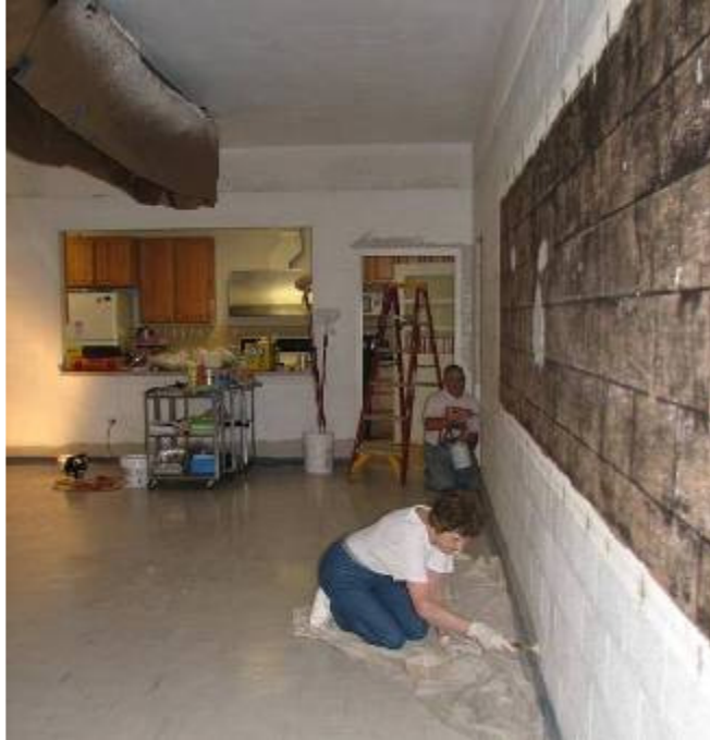
Lloyd and Marietta paint trim in the Wesley Foundation Fellowship Hall.
