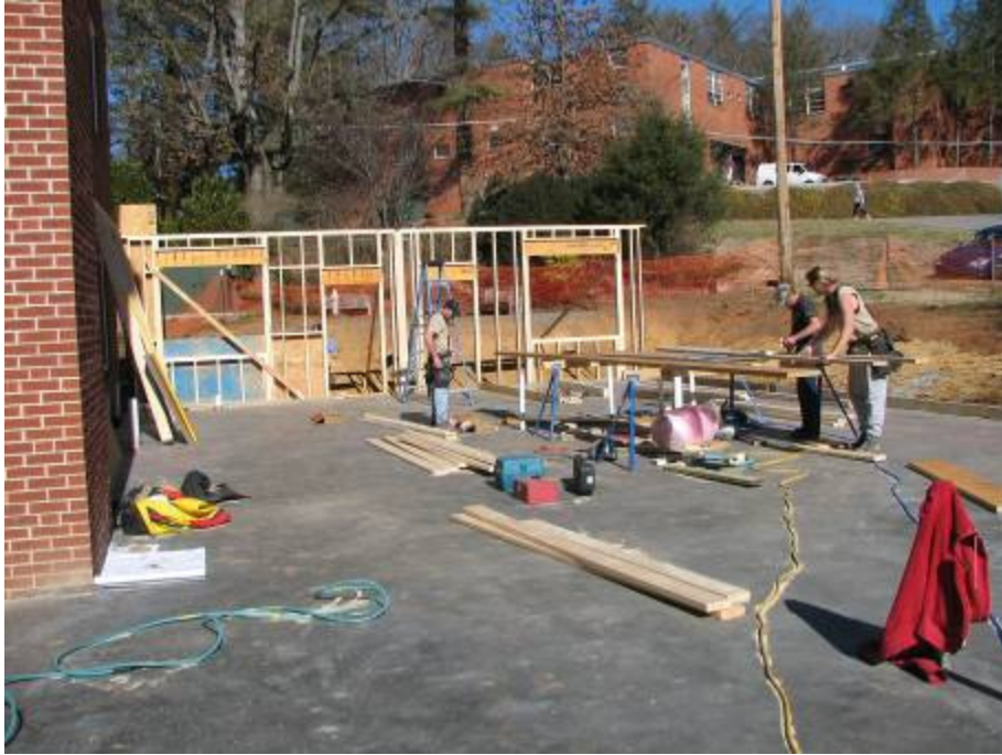
Day One of Framing
