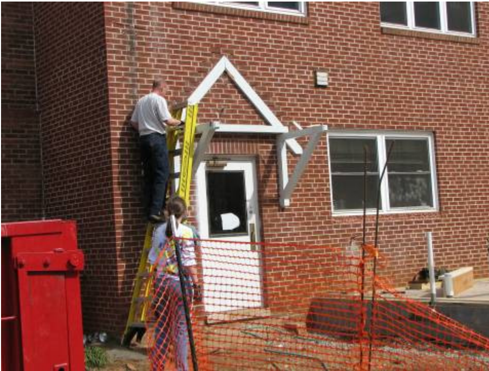
Demolition is always fun.
