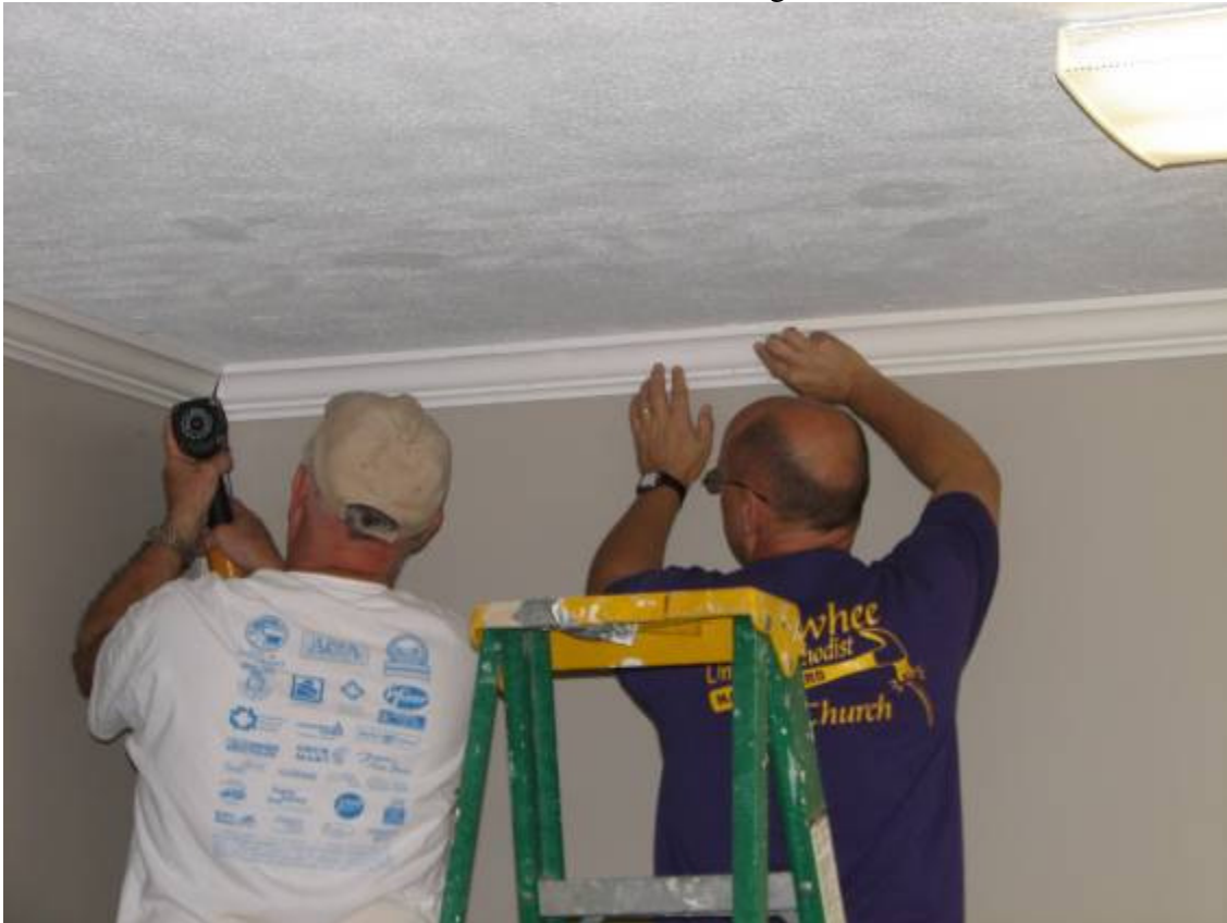
Earl and David install crown molding in the office.
